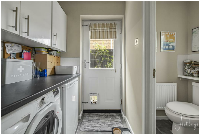
Plumbing for washing machine, tiled flooring, radiator.
